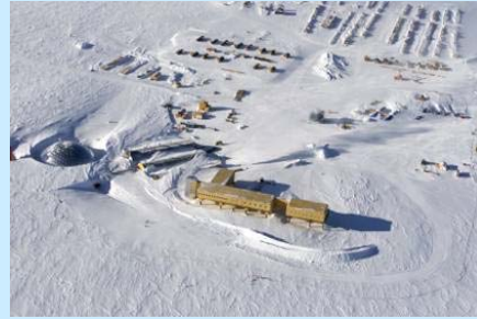
South Pole Research Station Established
